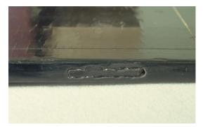
Fig. 8.18. Detail, screen (B67M8+), showing wood filling old hinge holes and groove.
